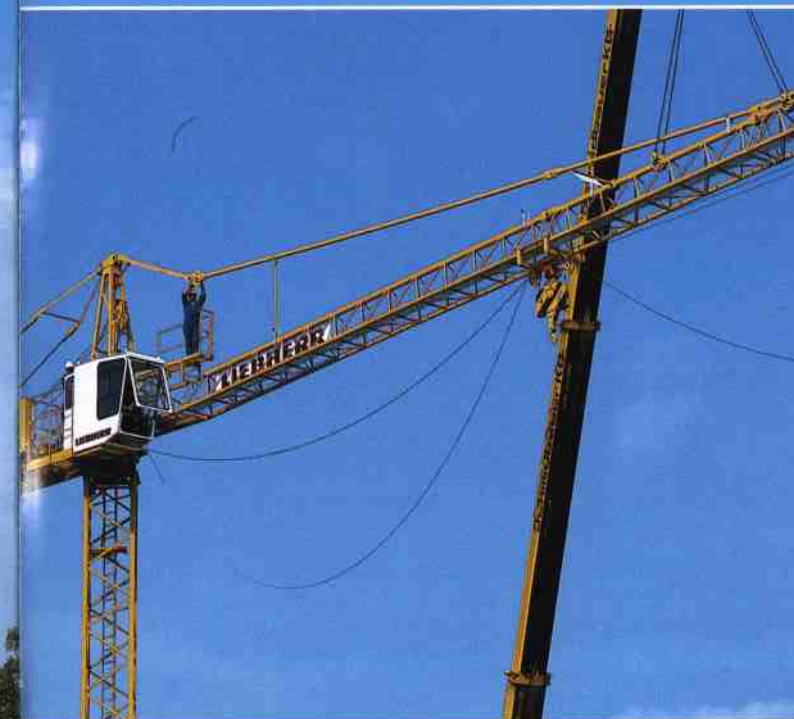
Working from a safe place, the jib tie-bars are connected.
