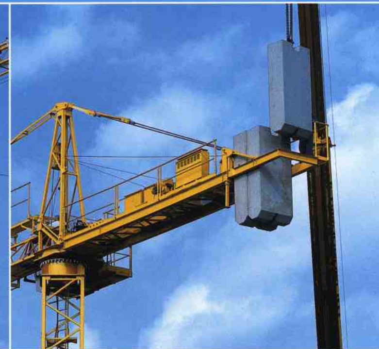
The rest of the counterweight is attached.
